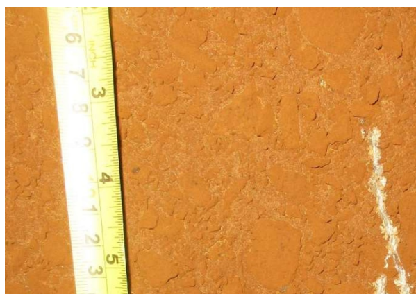
Fig. 2. Siliceous aggregate left standing proud.
