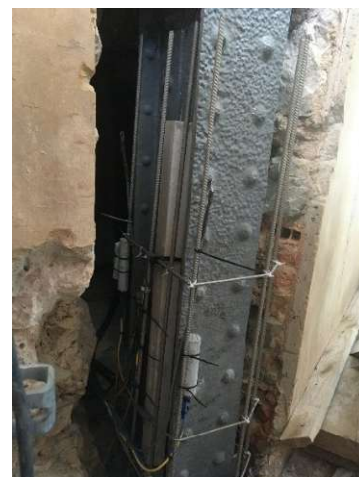
Fig. 5. Anode and RE placed along the steel column
