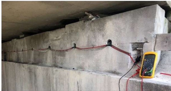
Fig.18. Treatment of the abutment using discrete Zinc 95 cm drilled-in anodes
