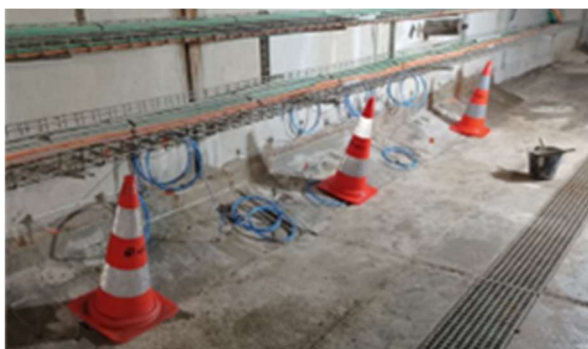
Fig.10. Pilot test in the tunnel ventilation gallery
