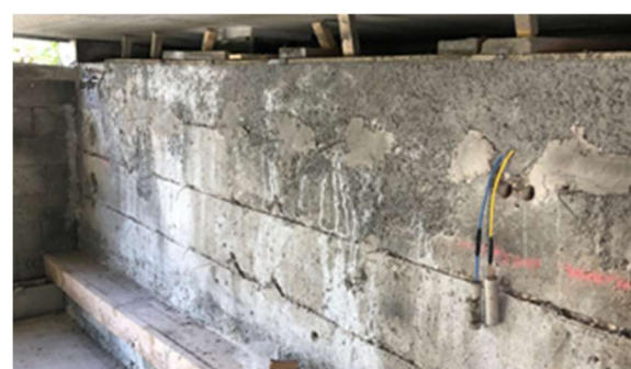
Fig.16. Treatment of the abutment using TiMMO discrete 950 mm drilled-in anodes
