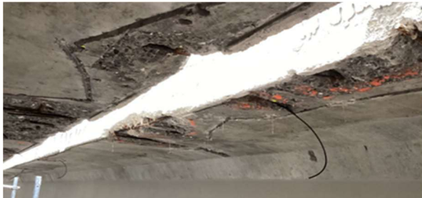
Fig.23. Installation of discrete drilled anodes around repairs
