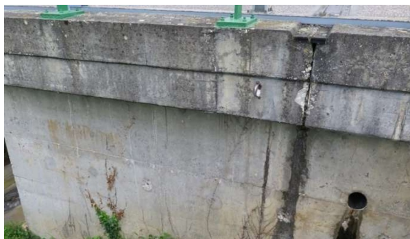
Fig. 2. Closed expansion joint.
