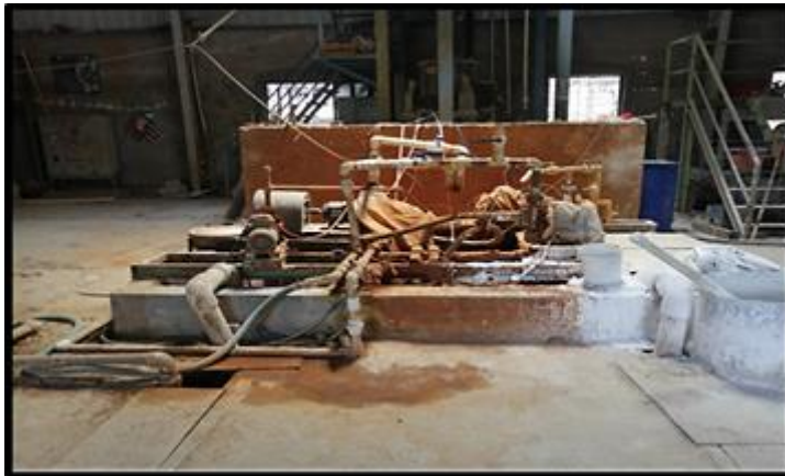
Fig. 1. Wastewater Tank on which work was identified
