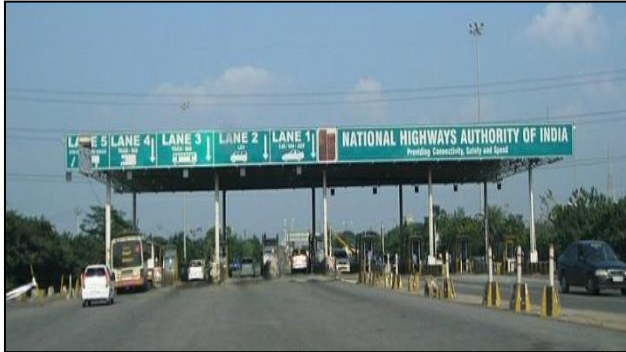
Fig. 6. Nemili Toll Plaza near Sriperumbudur
