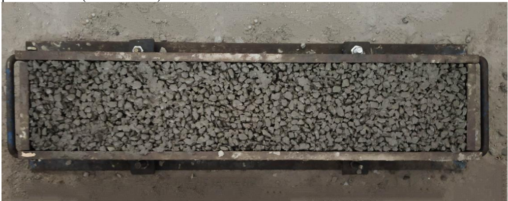
Fig. 5. Casting of beam
