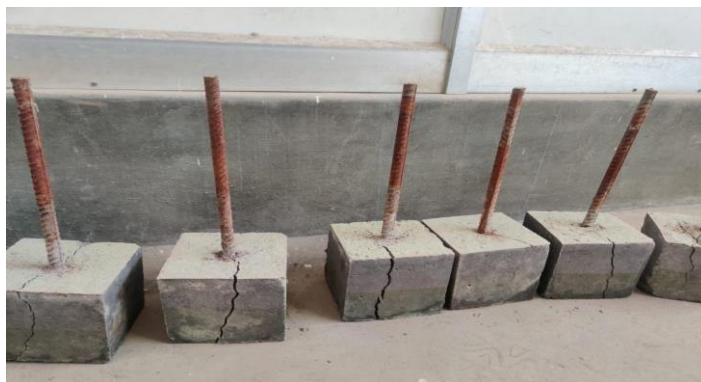
Figure 3: Failure pattern of specimen due to pull out test
