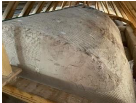
Fig. 20. Fiberglass and aramid nets reinforcing the vaults.
