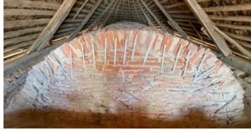
Fig. 19. Stitches of galvanized wrought iron fixed on the vault above the naos.
