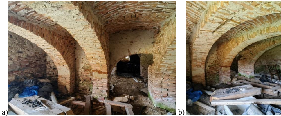
Fig. 8. Parish house: a) brick vaults over the basement; b) tie rods.
