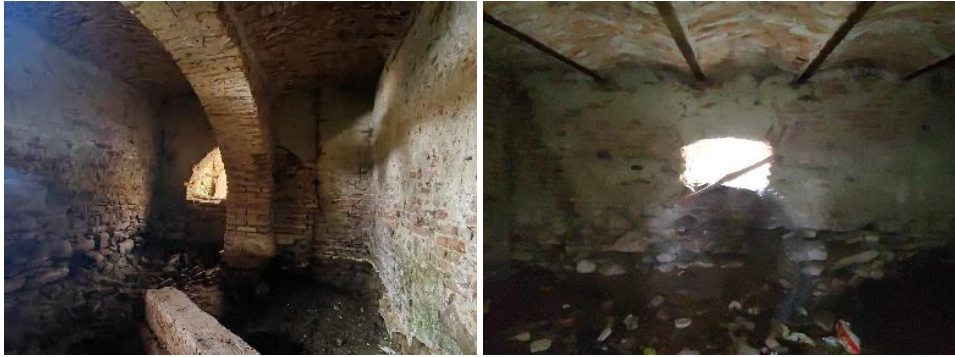
Fig. 12. Excavation of the earth from the basement.
