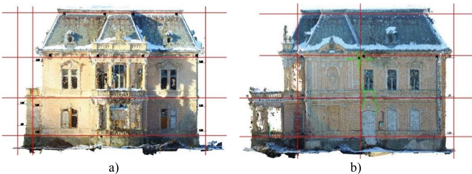
Fig. 10. (a) The main façade, (b) The right lateral façade.
