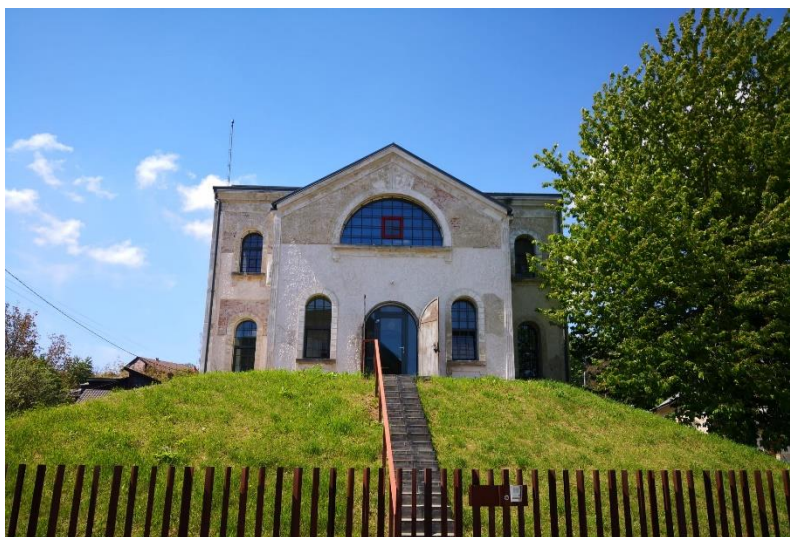
Fig. 10. The Old Suceava Water Plant, personal archive
