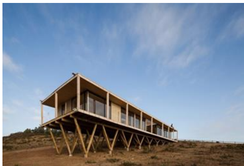
Fig. 15. The Dock House is located in the town of Pichicuy in Chile's Valparaíso region.
