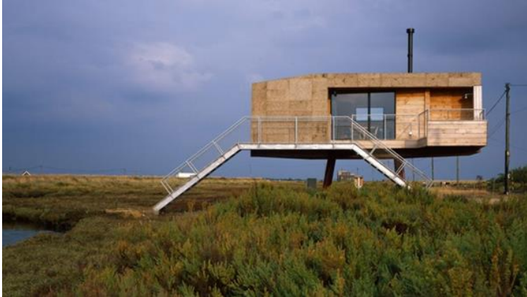
Fig. 9. Untreated oak boards and cork panels protect this cross-laminated timber, Redshank, UK.
