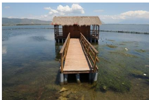
Fig. 4. Traditional stilt house “pelada” in Mesologgi Lagoon area, Greece.
