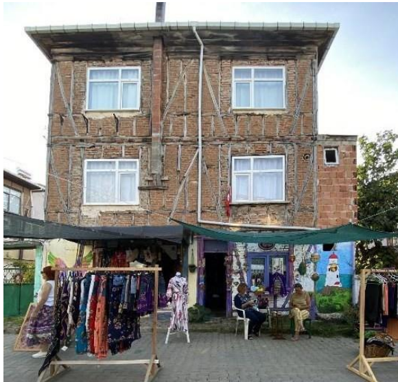
Fig. 2. Weekend use of the ground floor shops.
