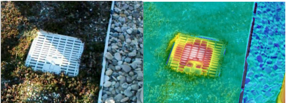
Fig. 6. Thermovision of the roof drain. [author]
