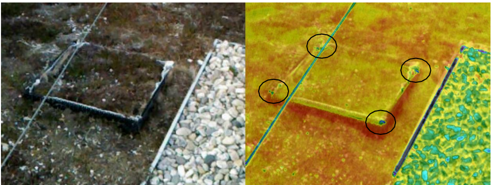
Fig. 7. Thermovision of the control segment. [author]
