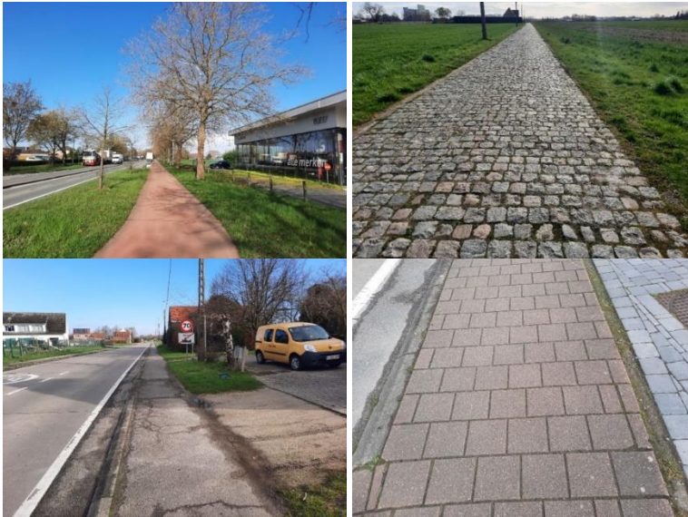
Fig. 2. Examples of sections to be used for the panel tests: a burlapped cement concrete bicycle path (upper left), a road with cobble stones often used by cyclists (upper right), a bicycle lane with a dense asphalt concrete (worn, lower left) and a bicycle lane in 20 cm x 20 cm cement concrete sets in fairly new state (lower right)
