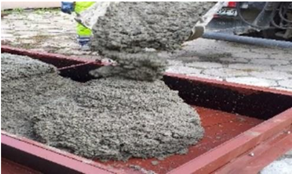
Fig. 7. Concrete mix with steel fibres during unloading into moulds.
