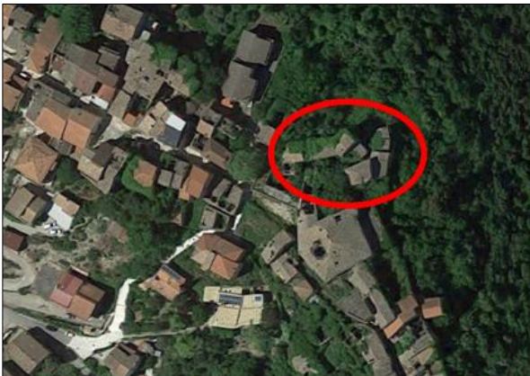
Fig. 2. Individuation of the masonry compound under study
