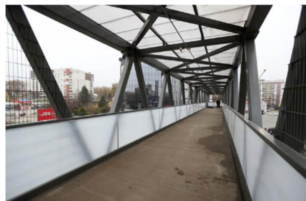
Fig. 5. Pedestrian bridge on the April 15th str.
