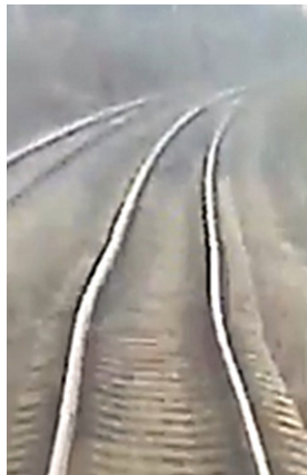
Fig. 4. Location of the rolling stock derailment
