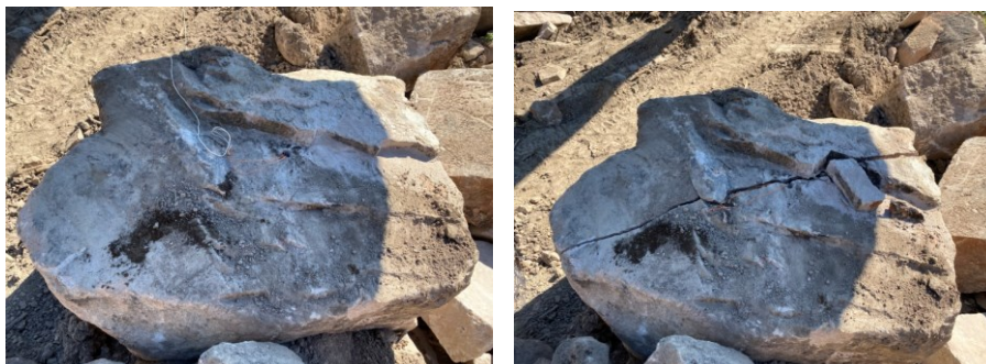
Fig. 2. Splitting of a boulder with one charge of 0,050 kg. Mixture #1 in single blasthole with length 0,60 m.
