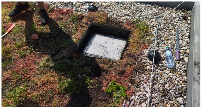
Fig. 6. Control segment installation.
