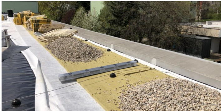
Fig. 4. Hydroaccumulation and gravel placement.
