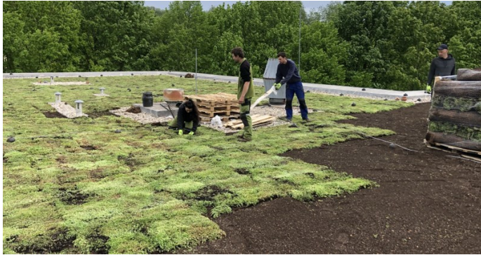
Fig. 5. Substrate and green vegetation carpet placement.
