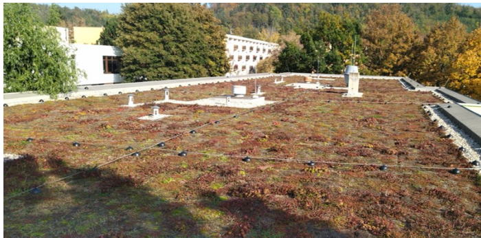
Fig. 8. Green roof in 10/2022.
