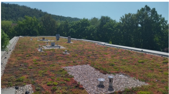
Fig. 7. Green roof in 07/2022.
