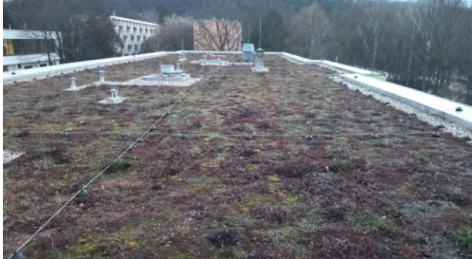
Fig. 9. Green roof in 02/2023.
