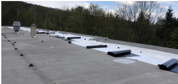
Fig. 3. Placement of geotextile and nop film.
