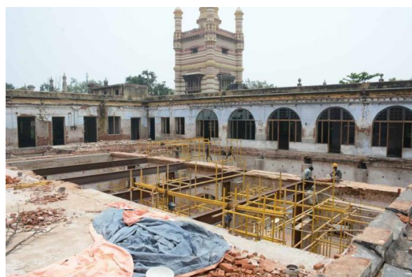
Fig 2. Renovation of the Structure during fire accident in 2016.
