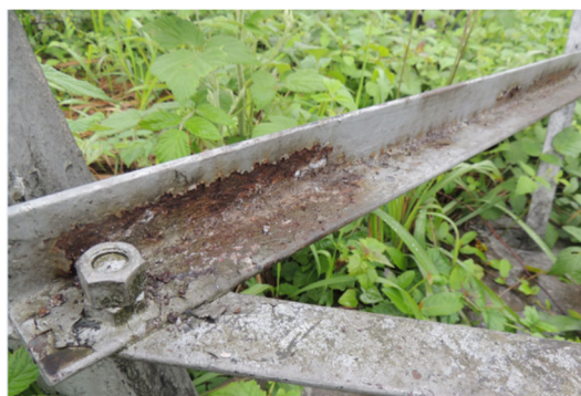
Figure 1. Local corrosion
