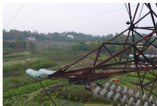
Figure 2. Uniform corrosion.
