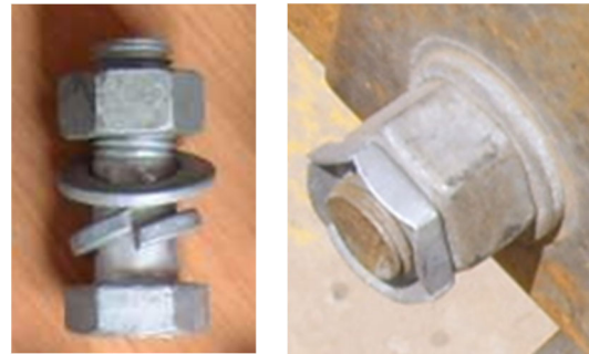
(a) Spring washer (b) Tightening nut
