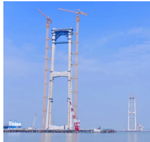
Figure 4. The construction situation on the spot
