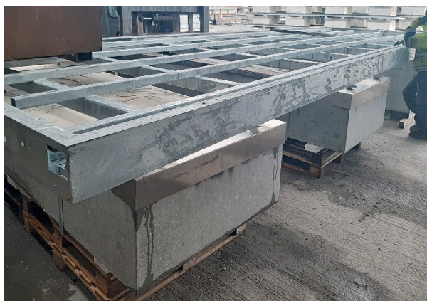
Fig. 8. Pre-assembled pontoon, in front the TR-UHDC floating units freshly mounted beneath the connecting frame.
