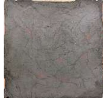
Photo3-3 Initial crack test results for Cu+PP fibers 0.05%
