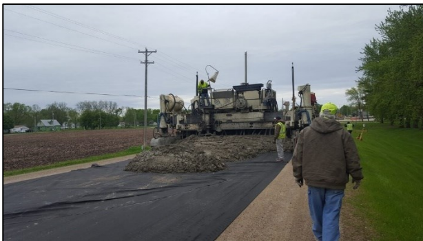
Fig. 12. Construction of a new COC-U overlay in Iowa over an existing COA-U overlay.
