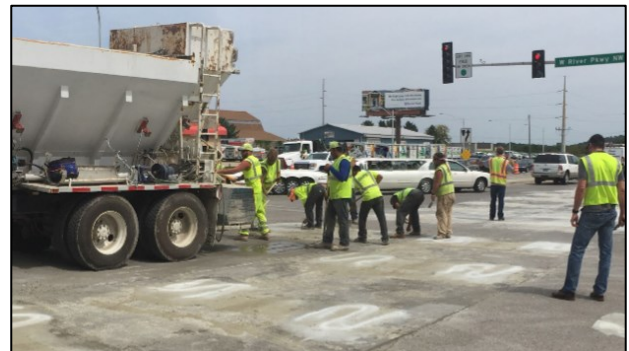
Fig. 5. Crew performing dowel bar retrofit on a COA-U pavement section in Minnesota [12].
