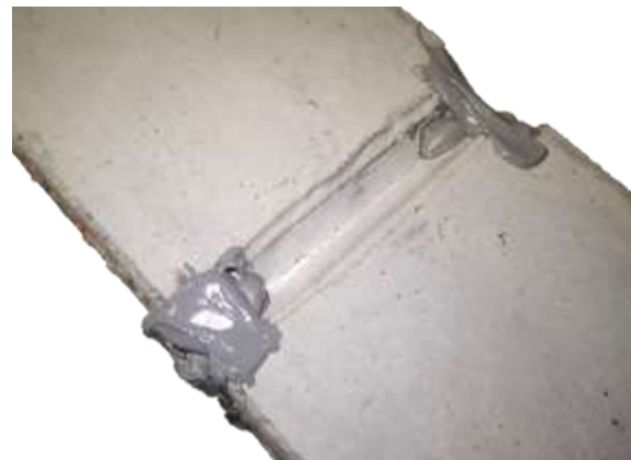
Fig. 3. Sample with separation crack
