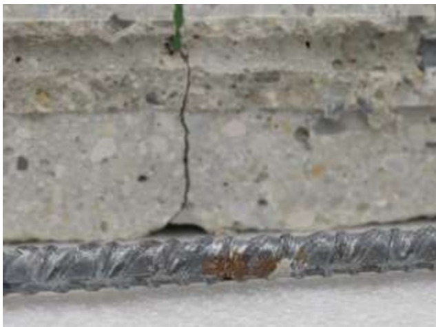
Fig. 7. removed black steel with corrosion in front of cracked concrete specimen
