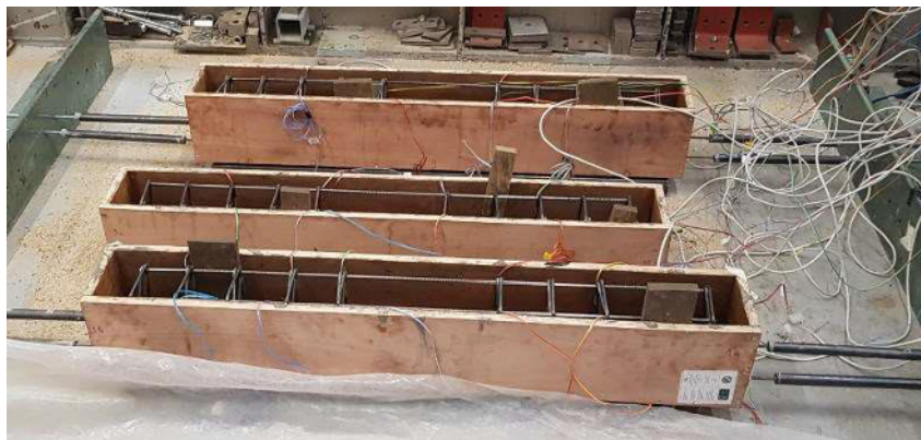
Figure 1 Prepared formwork and reinforcing cages in prestressing position. By Authors (2022)
