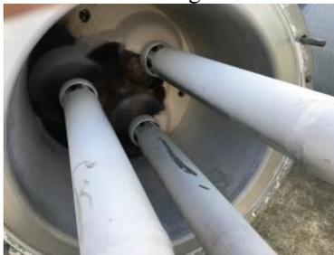
**Fig. 1** Vent basin insulator and conductor at fault side
