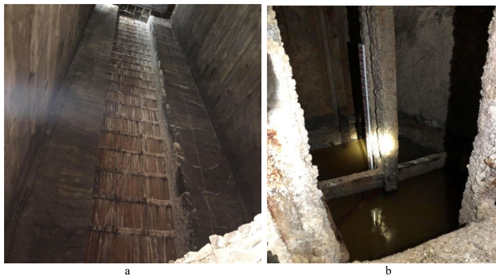
Fig. 3. a. Unirea Mine shaft; b. water level in the shaft sump, after 168 hours for it being drained
