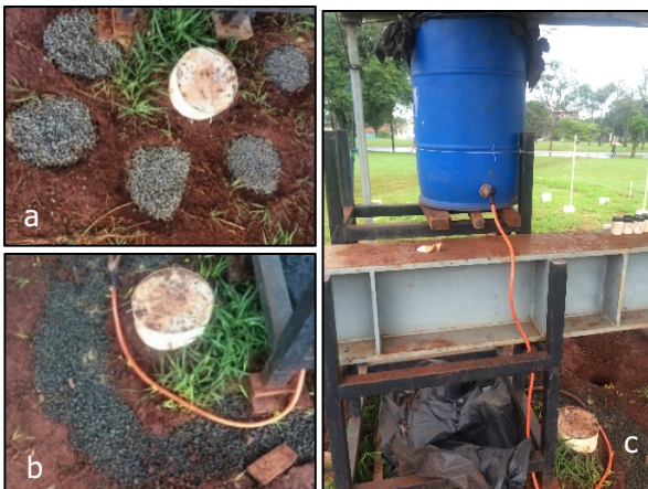
Fig. 2. Artificial pre-moistening setup. (a) Gravel-filled holes 40 cm in depth drilled around the pile; (b) Ring of gravels to cover the holes; (c) Water flowing around the pile through a hose.
