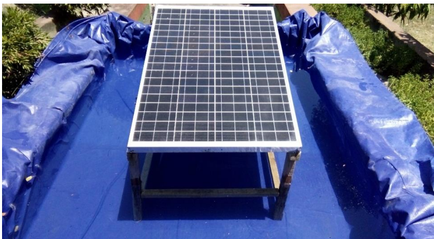
Fig. 1. Installation PV with floating cooling method
