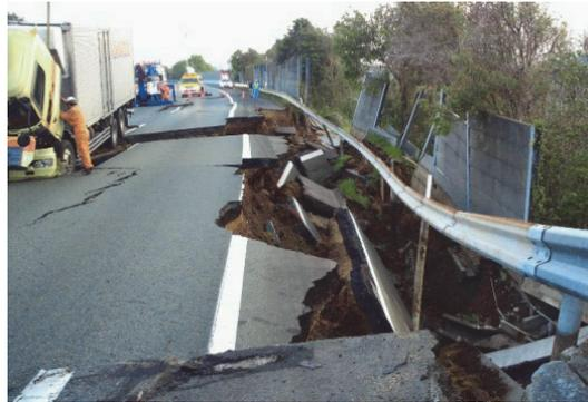
**Fig. 1.** Damage of road embankment during the 2016 Kumamoto earthquake.
