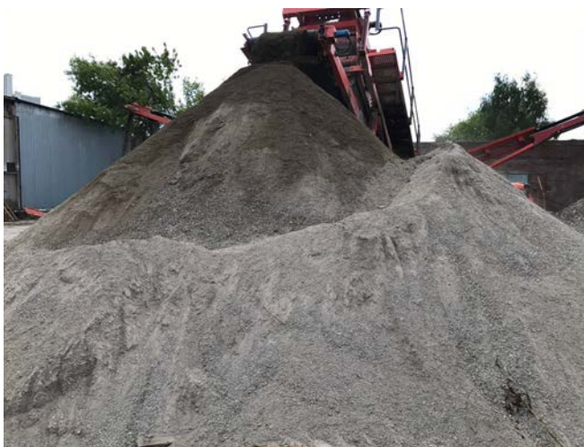
Fig. 4. Construction waste recycling (Lipetsk)
