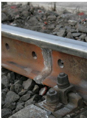
Fig. 1. Welded joint obtained by the aluminum-thermite method
