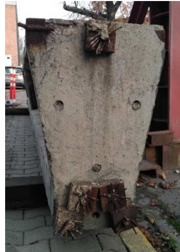
Fig. 3. Front view of the tested beam.
