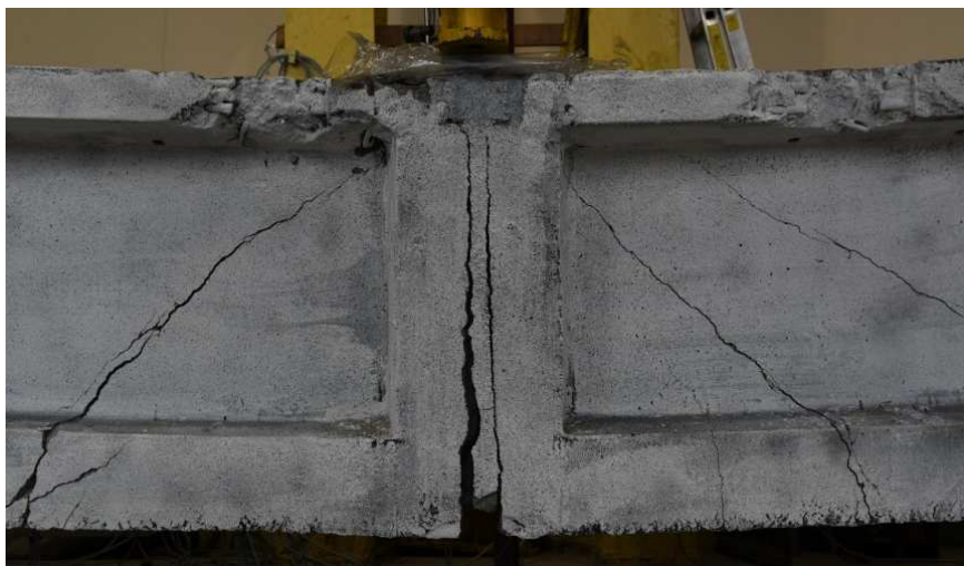
Fig. 7. Failure mode of KBP-03 specimen.
