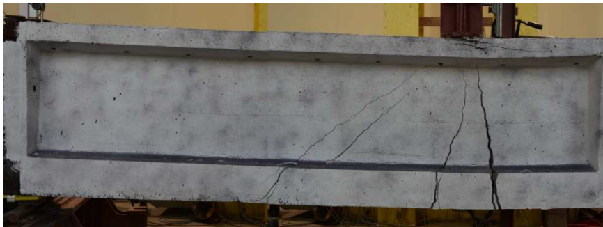
Fig. 6. Failure mode of KBP-02 specimen.
