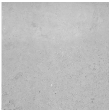
Fig. 1. Unevenness in surface coloration based on the example of a 10 x 10 cm section of concrete surface.
