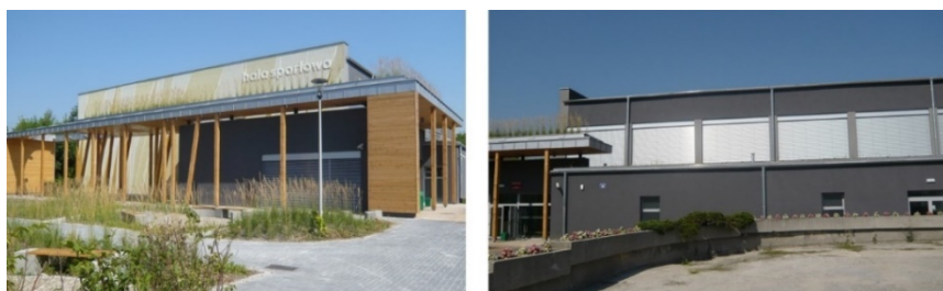
Fig. 1. Southern facade (left) and Eastern facade (right) (Author's archive)
