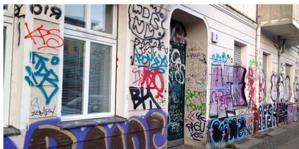
Fig. 1. House wall in Berlin [3]
