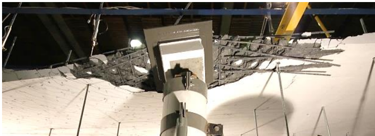
Fig. 8. View of bottom reinforcement bars – research of M. Wiczorek.
