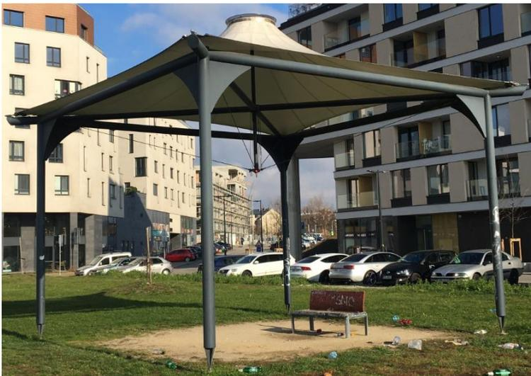
Fig. 2. Membrane structure in the shape of cone in Ostrava.
