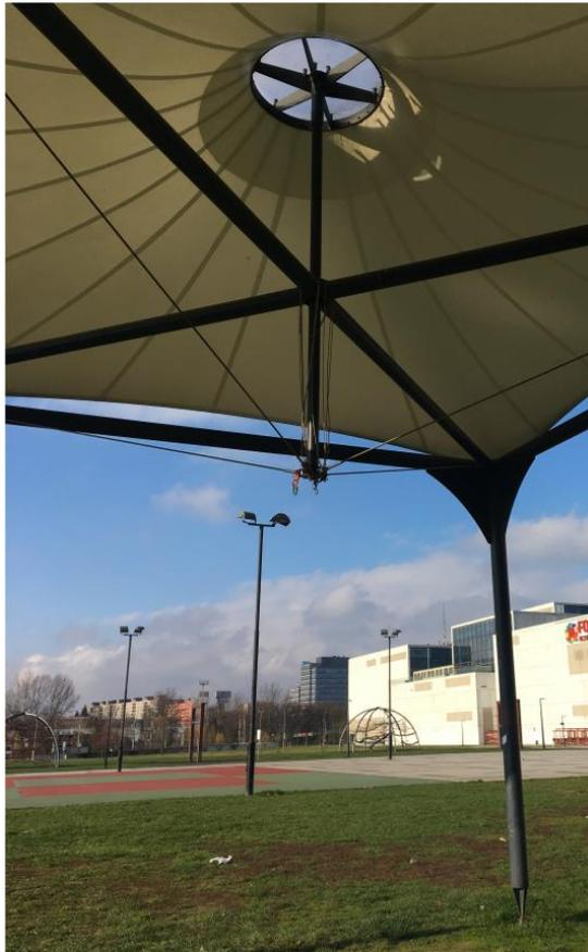
**Fig. 3.** Frame corner and system of rods to ensure rigidity of the structure.
