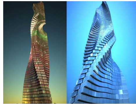
Fig. 3. Dynamic Tower Dubai
