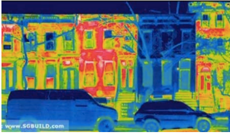
Fig 1. Thermal image of renovated to passive standards house next to neighbors without renovation (Photo: Sam McAfee of SGBuild)
