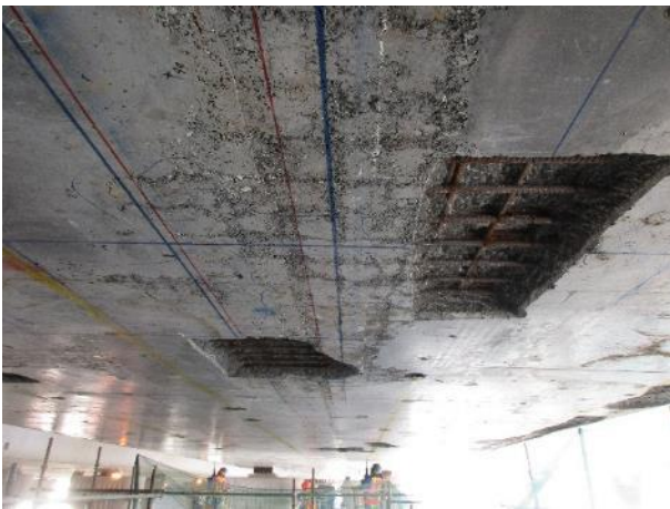
Fig.2. General condition of soffit
