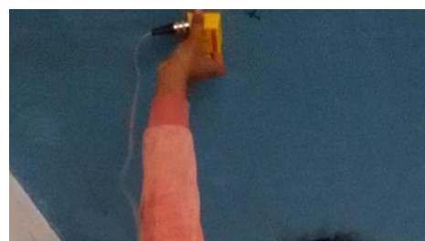
Fig. 5. Cover-meter measurement at the soffit of the roof slab.
