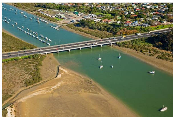
Fig. 1. Aerial view of the existing Whau River Bridge, looking south-west (Corbett & Watterson, 2016 [6])
