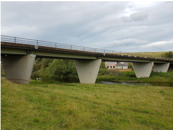
Fig. 3. Whiteadder bridge, Scotland, taken 10 years after installation
