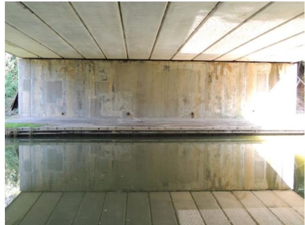
Fig. 4. Abutment shown from opposing bank 4 years after patch repairs
