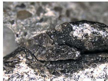
Fig 9. An example of detected cracks caused by JH.
