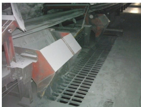
Fig. 4. The conveyor belt and charging opening.
